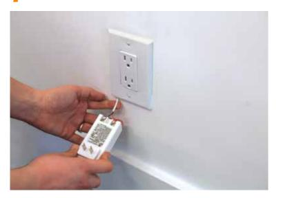
Gently pull the power wire through the wall at the outlet end. You may need to remove your outlet cover to do this. 8
