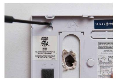
Remove the screws from the backplate of your panel and remove the panel from the wall. Please note there will be a small hole in the wall.
