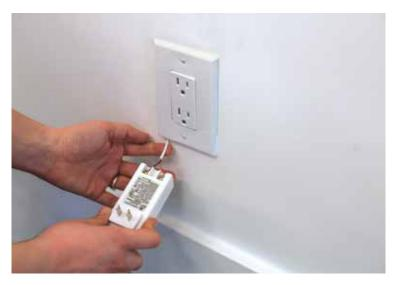
Gently pull the power wire through the wall at the outlet end. You may need to remove your outlet cover to do this.
